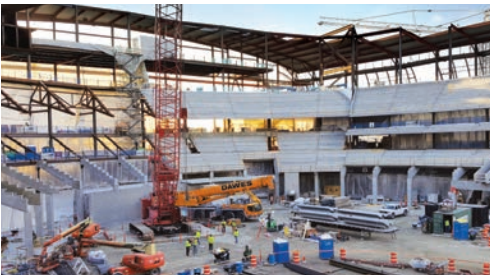
Installation of Spancrete risers at the new arena in downtown Milwaukee.
